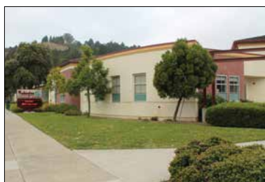
Washington Elementary School Point Richmond, CA ED Site Office
